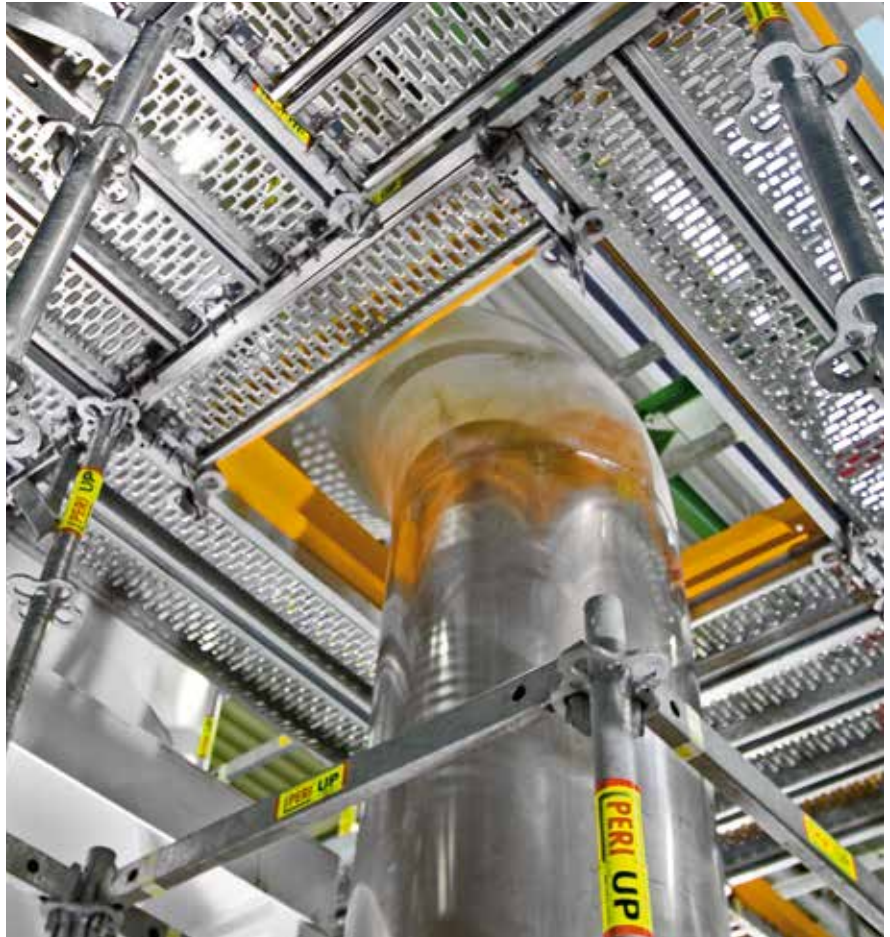
The change in direction of the decking in the 25-cm grid provides an enormous adaptability – and without any tube couplers.
