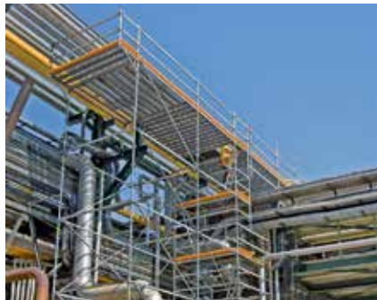
Workplaces for installation and maintenance work are quickly realised with PERI UP Flex. Pipelines can be easily accommodated and decking only installed where it is actually required.
