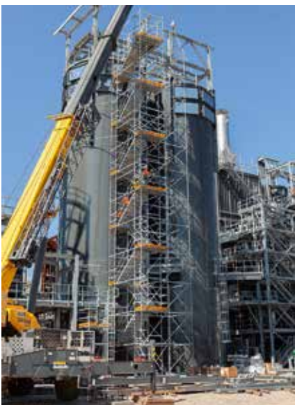
Stair towers with alternating staircase units provide greater head clearance and shorter walking distances for site personnel between levels.
