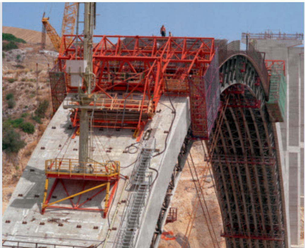
Section of the climbing scaffold with retracted formwork and climbing device.
