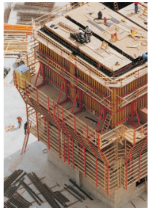
Photo (top): Completely enclosed building edges with PERI RCS.
