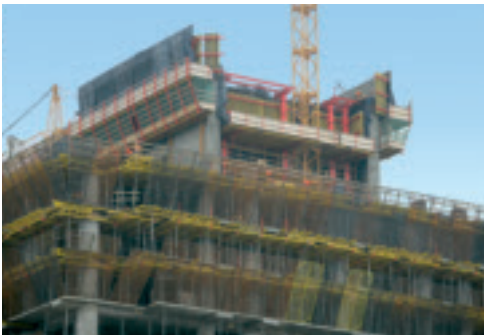
The use of the ACS system and VARIO, SRS circular column formwork, TRIO column formwork as well as PERI table modules was expertly synchronized to ensure construction progress was accelerated.
