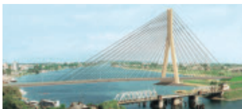
Through the new bridge, the infrastructure in the region around Gdansk – located on the Baltic Sea – has been significantly improved.
