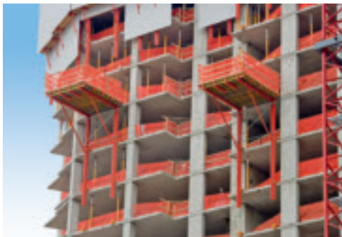
Landing platforms consisting of standard components for moving the slab formwork.
