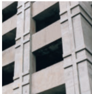
High quality standards were achieved for the in-situ cast facade.
