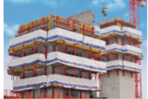
Bankside 123, London, Great Britain RCS Formwork Scaffolding on the building's core.
