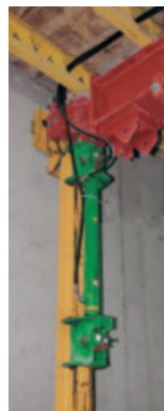
ACS 100 climbing mechanism with platform cross-beams and suspension of the finishing platform.
