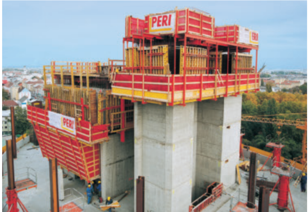
Both core groups climbed the floor slabs three and four storeys ahead in each case. All formwork units are movably suspended on a gallows frame.
