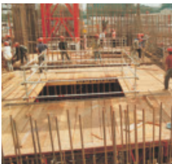
Photo (top): two of the three longitudinal external formwork units have already been raised and are now in position for the next cycle.
