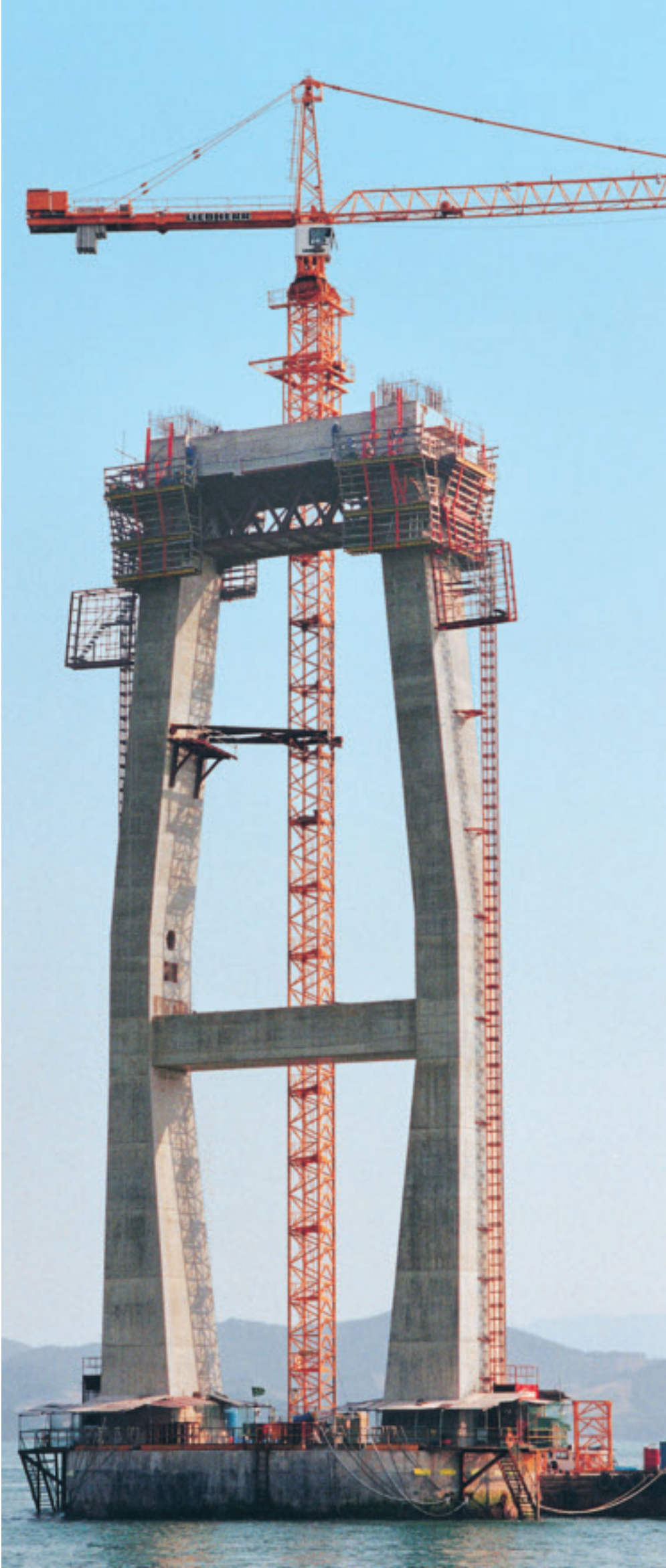
Section above the second cross-beam. ACS with modified platforms climbs unhindered past the cable sleeves that accommodate the stay cables.
