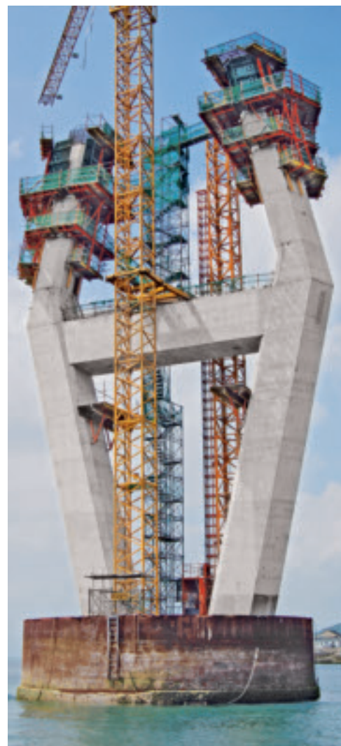
Geo Geum I: For forming and concreting the cross beams, the PERI steel framework construction transferred the loads reliably and safely into the structure.
