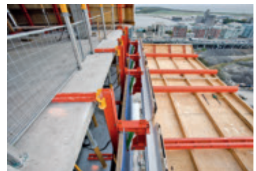
Hydraulic hinged units of the climbing protection panel for extending large-area slab tables such as the PERI SKYTABLE.
