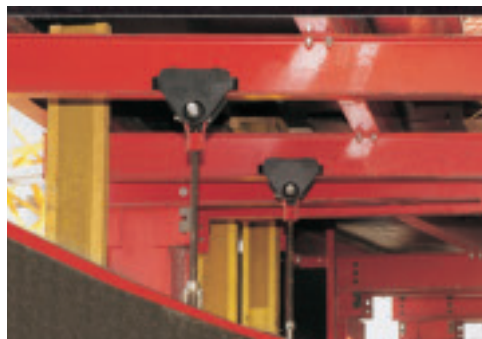
Formwork suspended on the gallows with height adjustment, movable on manually-operated carriage.
