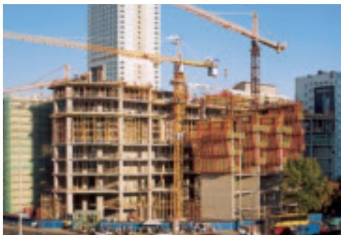
ACS, VARIO, SKYDECK on MULTIPROP towers, SRS, TRIO and the climbing protection panel cost-effectively combined.
