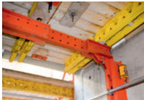
RCS shaft solution: as a platform beam, the RCS climbing rail can be continuously telescoped.
