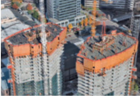
Bellevue Towers, Seattle, USA ACS P and G versions for the core, RCS climbing protection panel on the facade.
