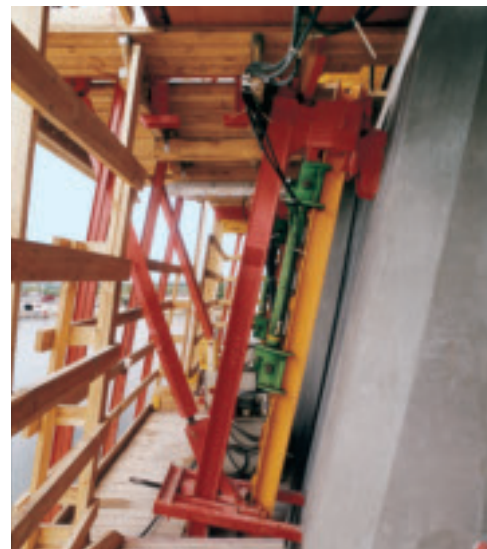
With 100 kN lifting force per bracket, the ACS climbing system has numerous safety reserves. The ACS 100 climbing unit with the patented rack system works automatically, safely and without any jerky movements. It has a climbing speed of 0.5 m/min.
