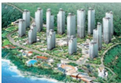
On the 50,000 m 2 area, a total of 15 multi-storeyed buildings, ranging from 70 to 150 metres high, have been constructed.
