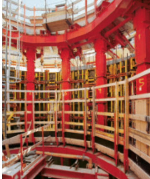
The core wall was formed with PERI GRV articulated walers and externally using PERI RUNDFLEX formwork. Adapting to the changing wall thicknesses was carried out with filler elements on the external formwork.
