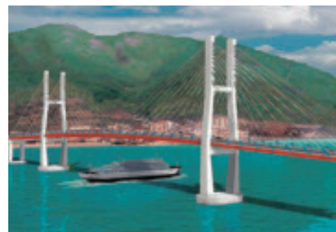
Artist's impression of the finished bridge: 30 m of clear headroom allows the passage of ships of up to 5,000 t.
