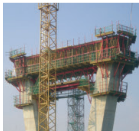
Geo Geum I: For forming and concreting the cross beams, the PERI steel framework construction transferred the loads reliably and safely into the structure.
