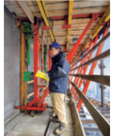
Using a remote control, three ACS platforms could be easily and safely moved at the same time.
