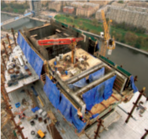
The VARIO external formwork climbed on ACS R platforms in advance and thus provided effective wind protection for the reinforcement work.
