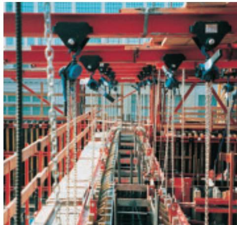
The internal wall formwork could be quickly and safely brought into position using chain blocks.
