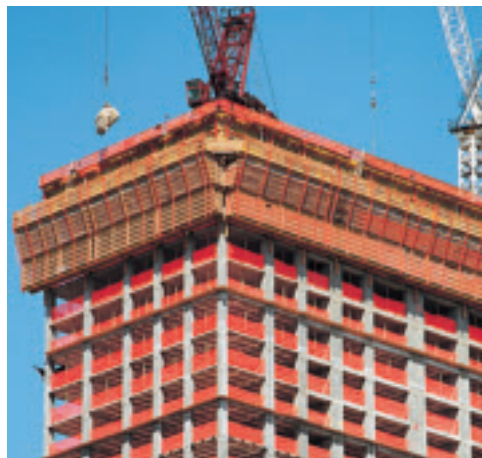
All platform levels are completely enclosed so that the personnel can work safely, secured against falling.
