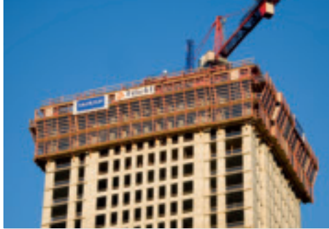
Kinsey Station, Chicago, USA Massive perforated facade with ACS R.
