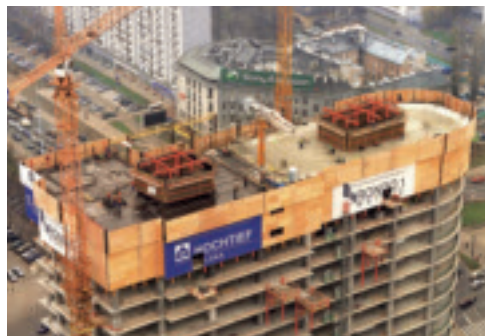
The PERI climbing protection panel provides personnel with extremely effective protection against falling and weather conditions. This naturally increases productivity levels.
