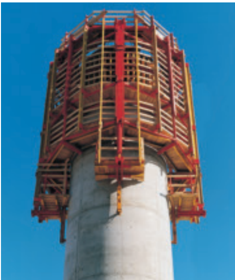
3.30 m high VARIO girder wall elements internally and externally were tightly coupled using VRK couplings. Special circular walings provided the exact shape required.
