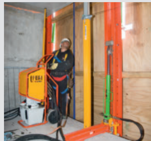
The hydraulic cylinder, with 5 t lifting capacity, can be easily positioned on the climbing shoe and rail.
