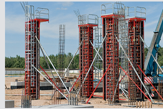
Column Formwork
