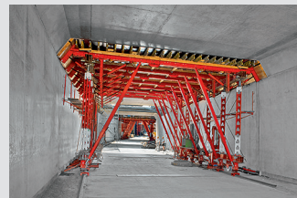
Tunnel Formwork
