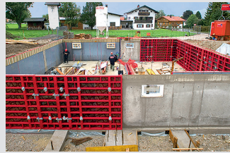
Wall Formwork
