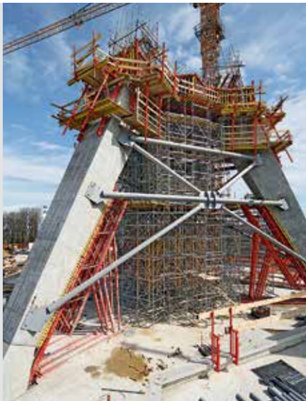
Same system components for providing temporary support for the structure as well as for climbing scaffold application.
