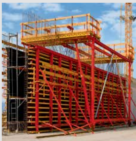
Clearly visible are the 2 separate concreting cycles, the wall on the left and the slab on the right. Both sets of formwork are designed as mobile units.
