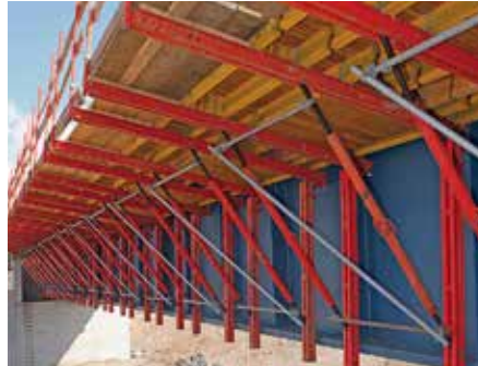
Bracing the bracket units with commercially available scaffold tubes Ø 48 mm.
