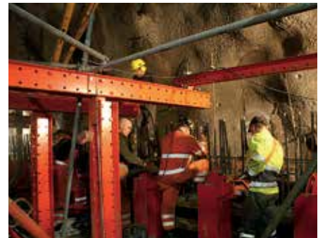
System components for the carriage and the movable formwork suspension allow flexible utilization.
