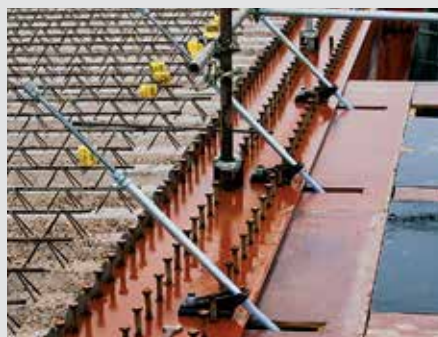
Anchor plate with pipe nut and DW 15 tie rod, can be operated from the top side of the bridge.
