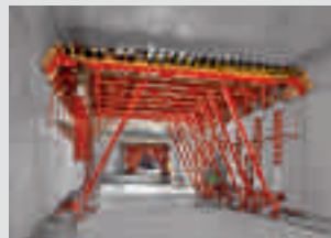
Tunnel Formwork
